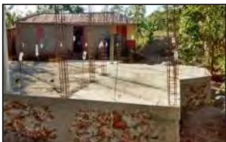
Thermy's foundation is completed and the blocks are made.
