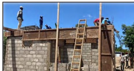
Etidieu's Walls are up; Next comes the roof
