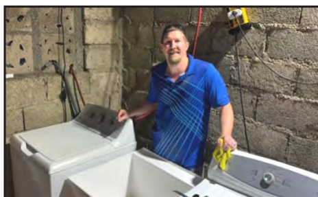
Austin installed an in-line pump for our friends
